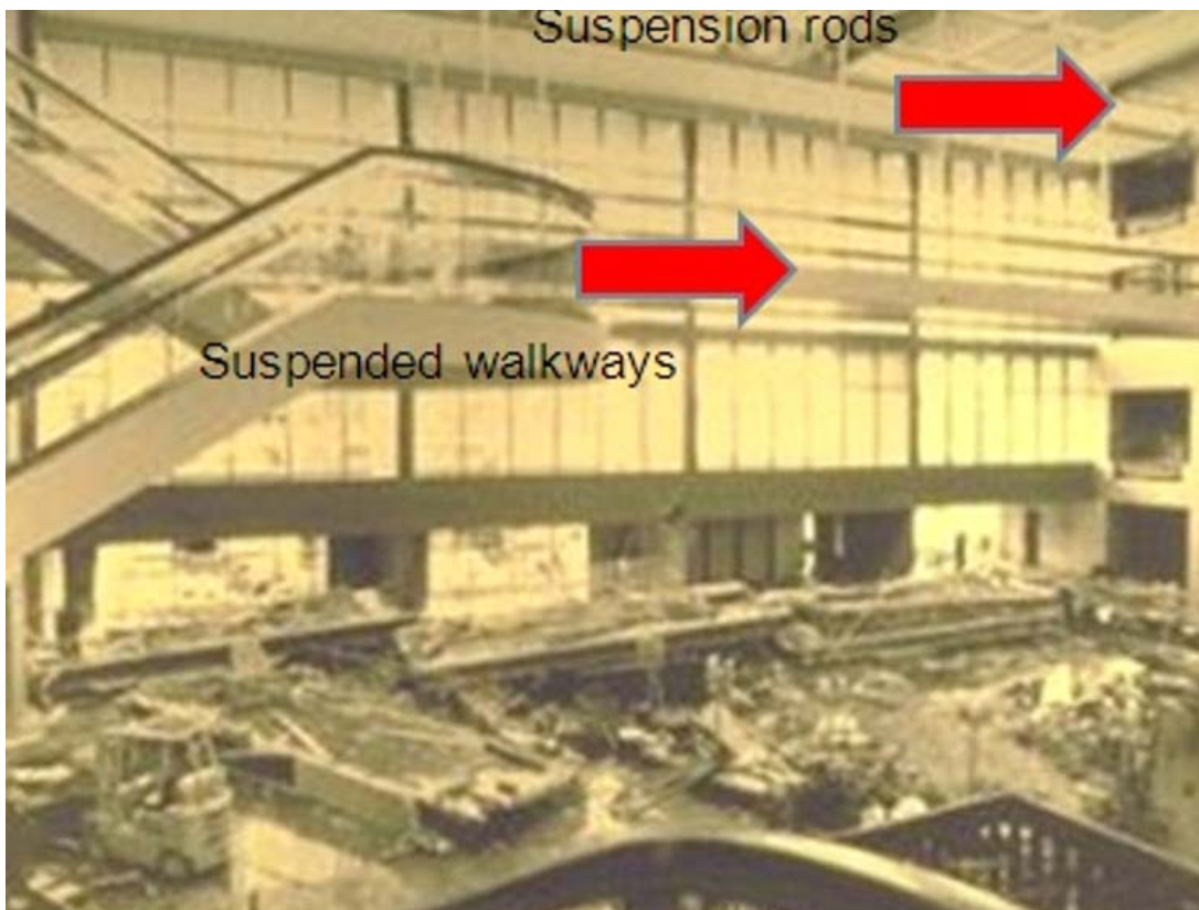
Figure 5 Suspended Walkways at the Atrium Lobby
